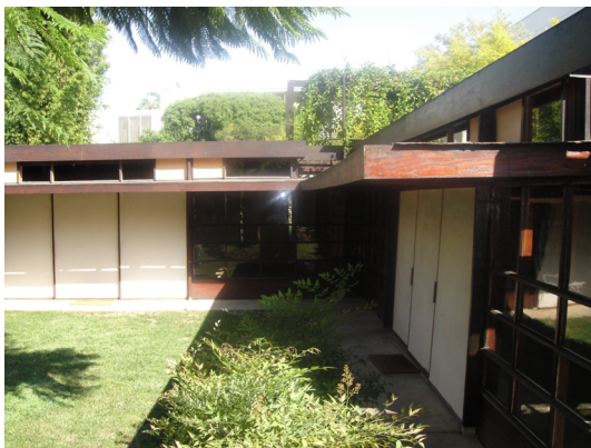
Fig.5. Clerestory Window over a Large Overhang
